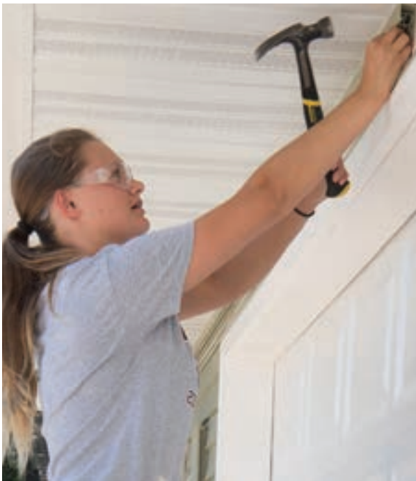
Indian Hills Community College construction technology student working on site.
